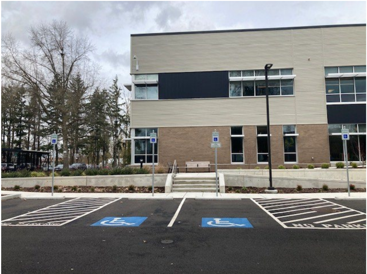
Parking spaces in front of LCDDS building. Access space next to each parking stall. Additional stair access leads to second level of ramp.
