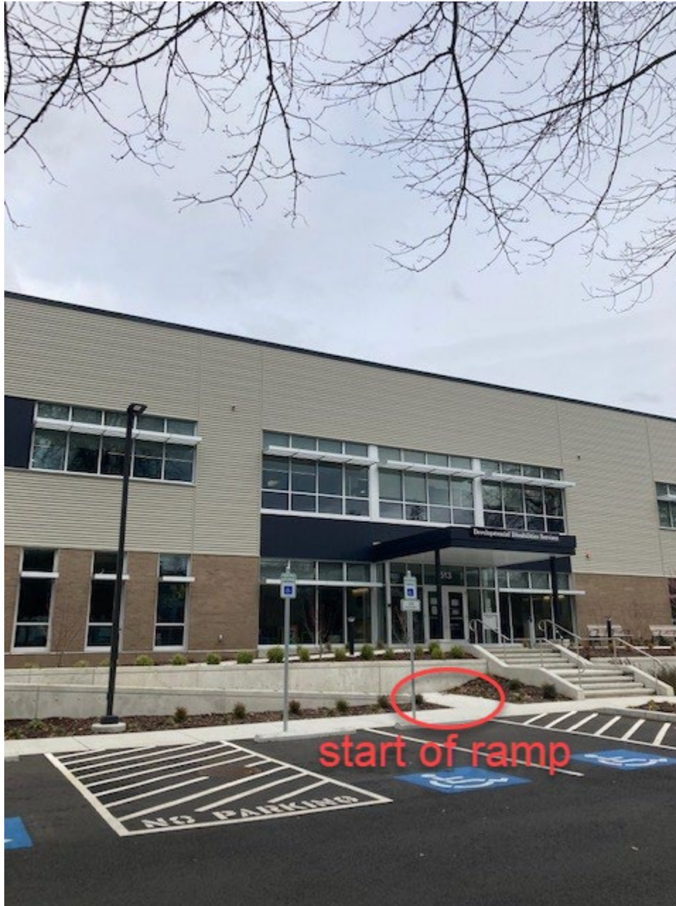
This shows the ramp entrance and main stair access to the front of our office. The ramp is a two level ramp for gradual incline.
