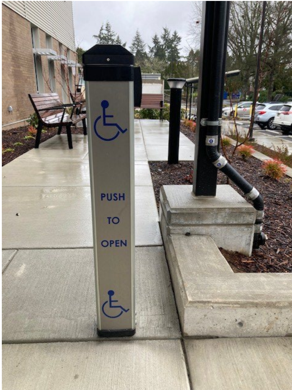
Automatic door button located at the top of the stairs and ramp (in front of main doors to building)
